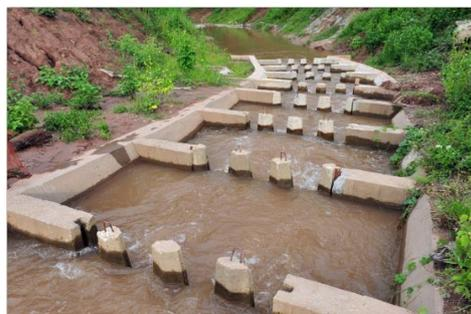
Gambar 1:3 : *Downstream Pak Peung Fish Passage* (MRC, *Mitigation of the impact of Dams in Fisheries 2017:27*)
