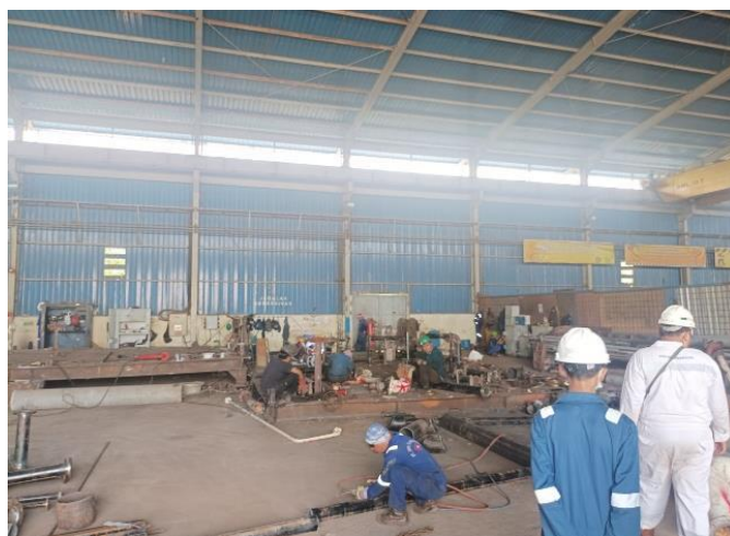
Gambar 2. 1 Piping Workshop Galangan SMI 2
